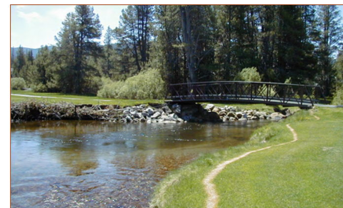
Several undersized bridges along this reach are located within the floodplain, constricting flow and accelerating velocities leading to erosion downstream.
